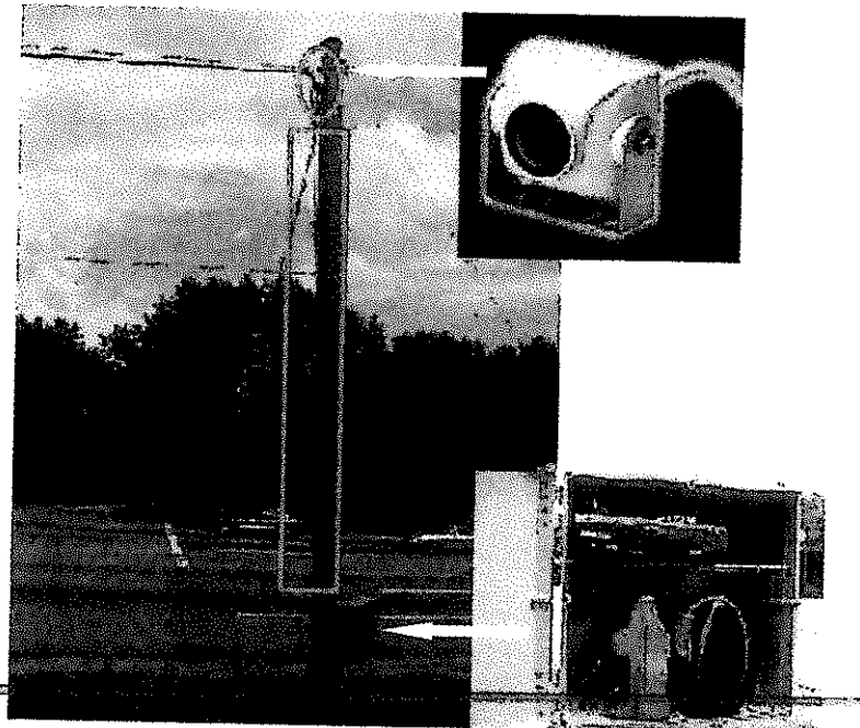
Figure 20 Camera and Equipment Cabinet Temporarily Mounted on Traffic Pole
