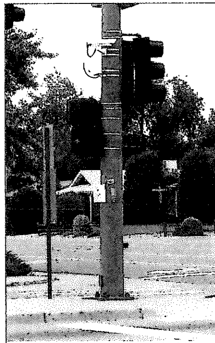
Figure 15: Non-intrusive vision-based signal phase detection systems (top camera) & presence detection systems (angled camera and 'presence view' below).
